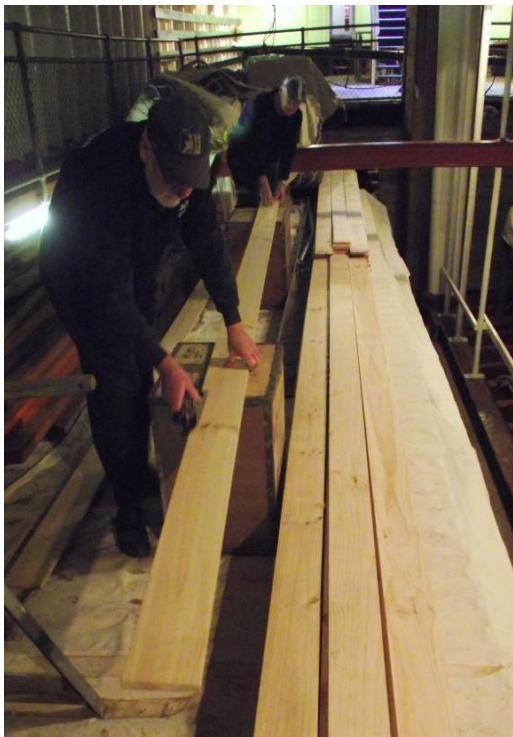
Photo 08 - Don Knowles planing edges of spar ceiling planking. Photo 09 - How it will look completed.
