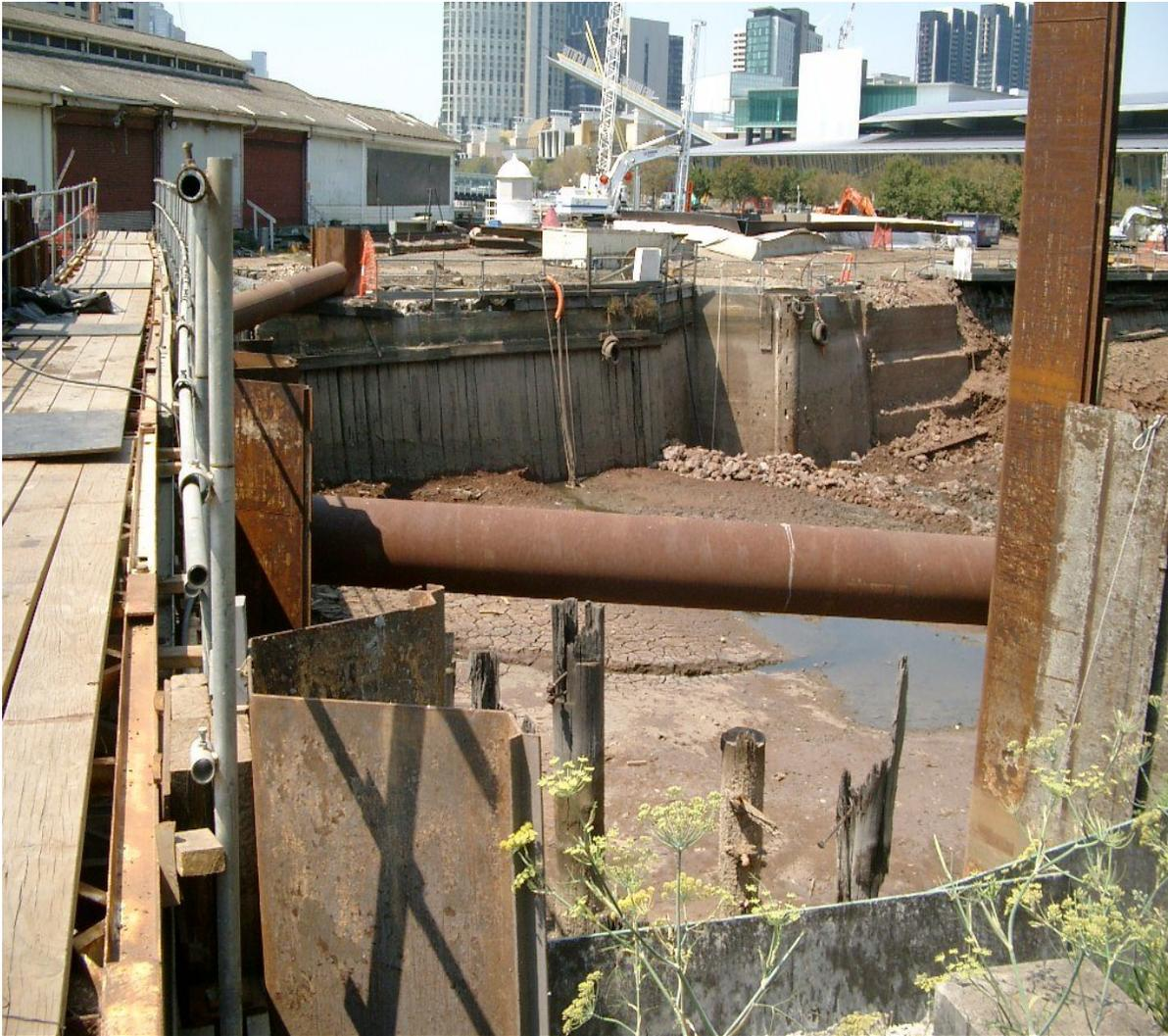
The Drydock is again dry (well more or less). This image was taken by Glen Stuart a couple of weeks ago and shows part of the “back-up” sheet piling suitably braced. Note the curve in the Bailey bridge due to water pressure. The river is to the left, Jeff’s Shed to the right.
